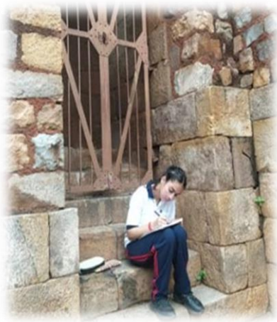
Within Allauddin's Tomb & Madarsa, where the iron door is kept locked leading to a staircase primarily for preservation to prevent damage and restrict public access.
